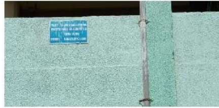
Image 8) Sludge dewatering unit
